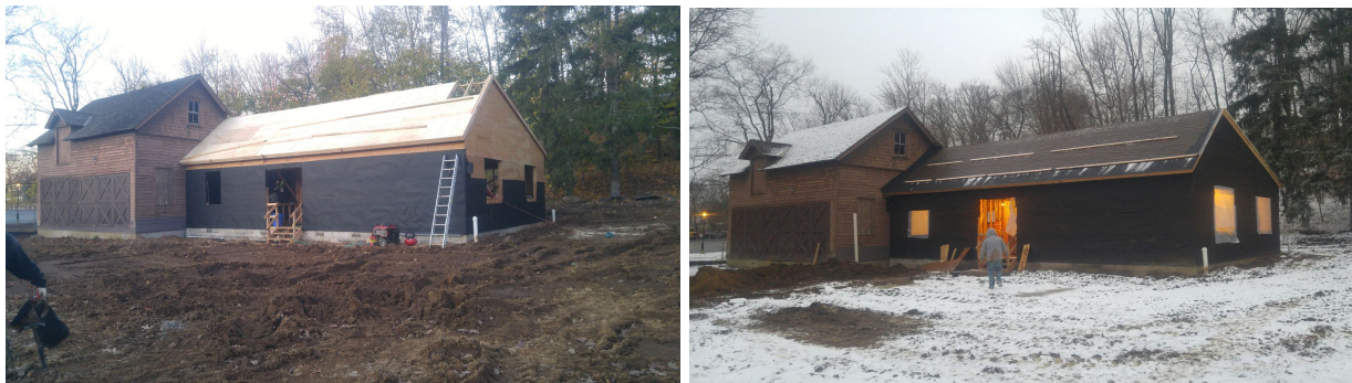
Above left: Nov. 10th, exterior wood sheathing applied
